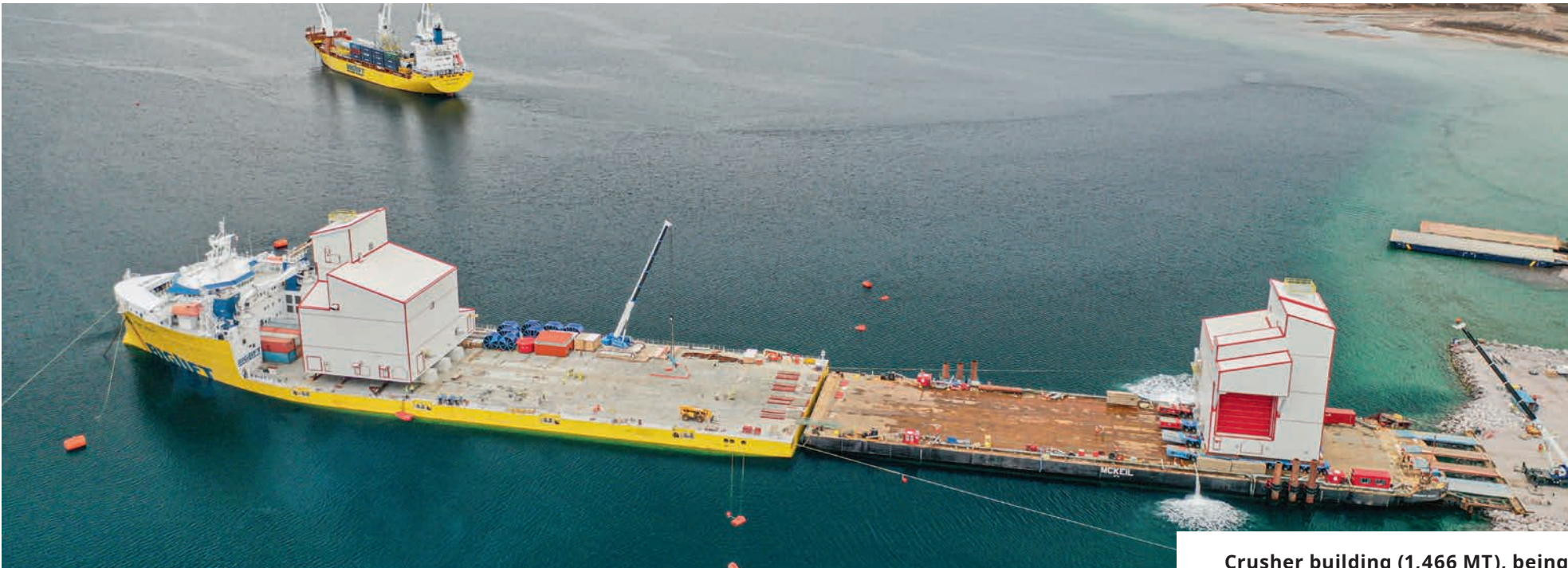
Crusher building (1,466 MT), being moved over the transition barge on four individual 16-axle SPMTs
