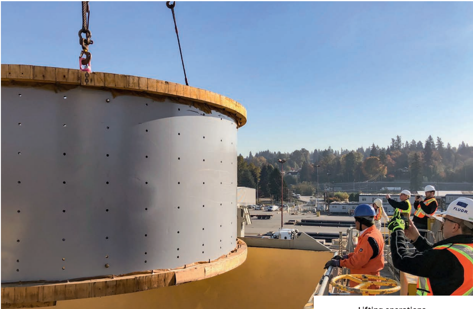
Lifting operations, involving a 35 MT shell with a diameter of 7 m, at the Port of Vancouver, Canada
